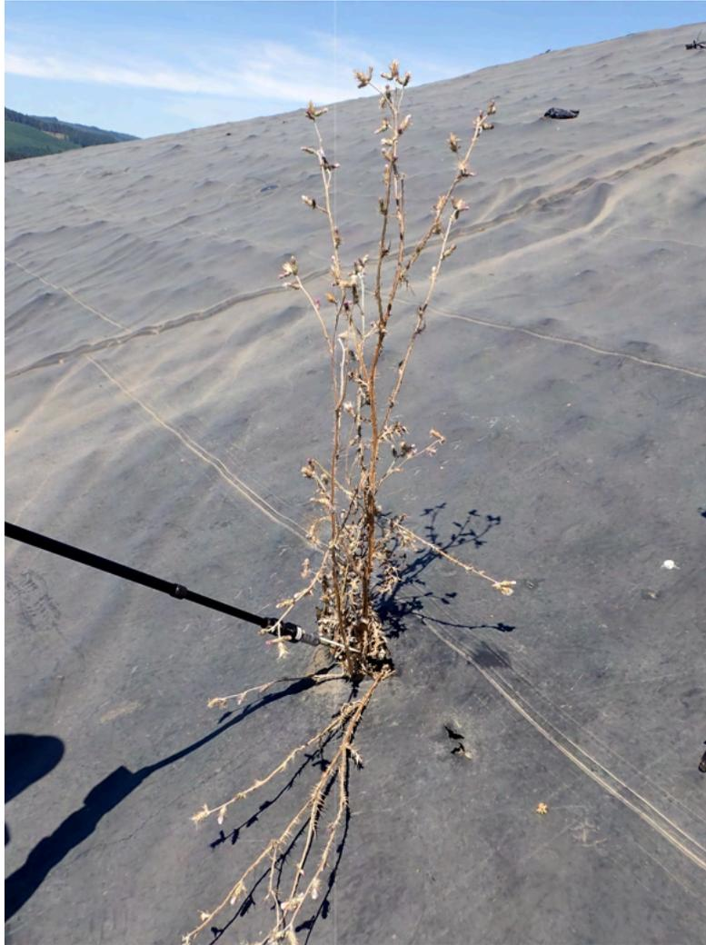
Caption: The EPA found multiple instances of vegetation growing through the tarp of the Coffin Butte landfill in both 2022 and 2024. The picture is one such example. The EPA measured methane at 1,000 ppm, twice the regulatory limit, near the base of the plant. Operators are supposed to constantly monitor the tarp integrity to ensure that there are no areas where methane could be leaking.
