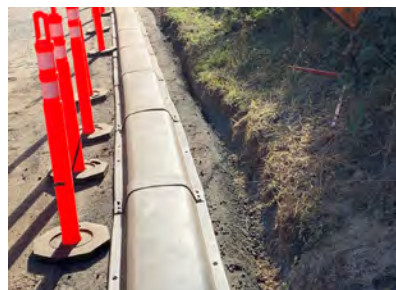
Cover installed over cable tray system
