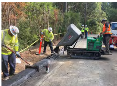
Geopolymer concrete pouring into tray system
