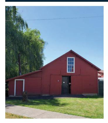
The Mentzner Machine Shop was observed to be in better exterior condition than most of the other buildings on campus. The major concern is the east roof, which is directly underneath a willow tree. The roof shows heavy debris from the tree, which provides potential to trap water and erode the roof surface (Figure 18.1).
