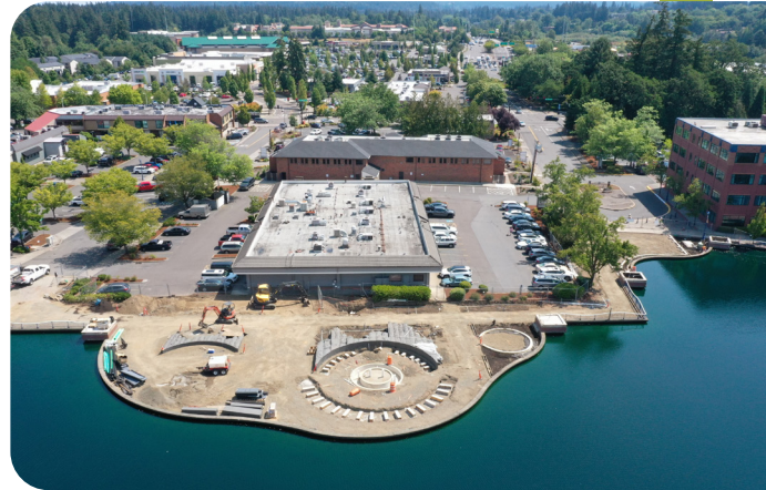
Veterans Plaza Under Construction, September 2024
