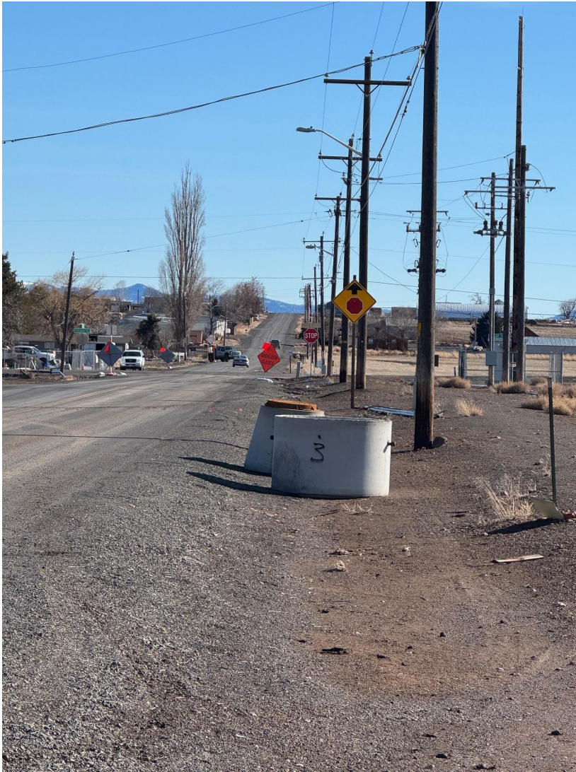
Manholes on-site and ready to be installed. Photo taken on 2.20.25.
