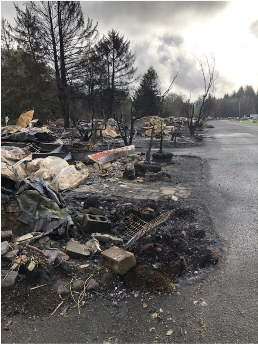
The Echo Mountain fire burned 29 of the 31 homes in the Salmon River Mobile Village on the north side of Oregon Highway 18.
