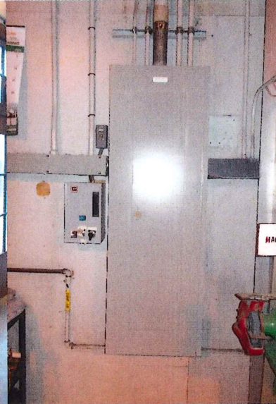
100 Amp disconnects for main boilers
