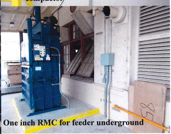
60amp fusible disconnect for compactor
