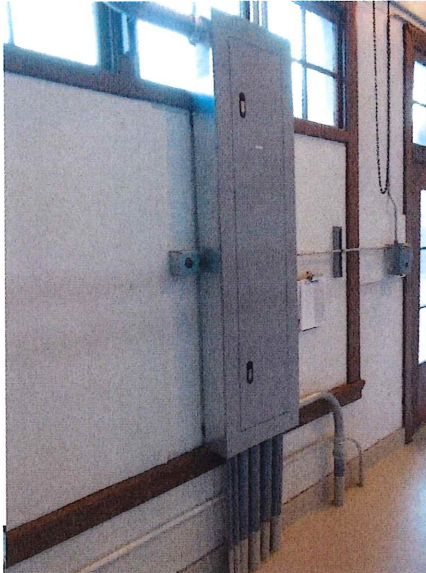
100 Amp disconnects for main boilers
