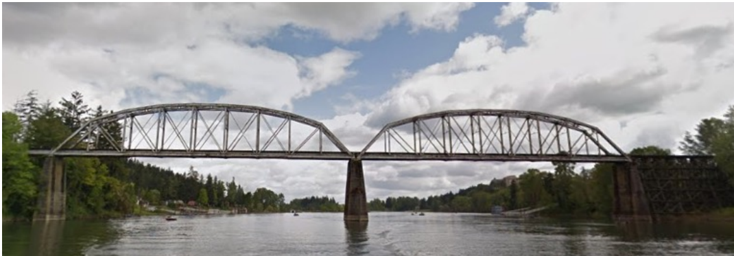
Oak Grove – Lake Oswego Railroad Bridge
