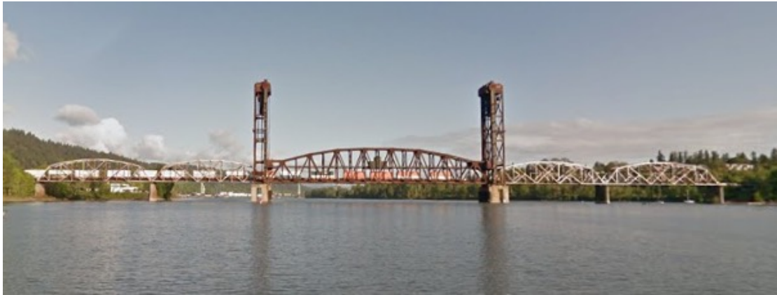
BNSF Railway Bridge 5.1
