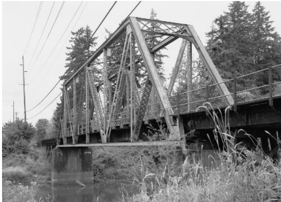
Tualatin Railroad Bridge – Milepost 35.3
