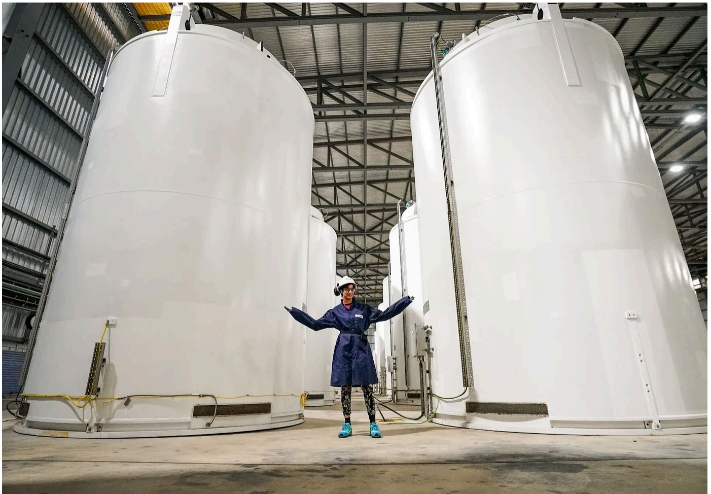
Visiting dry storage casks at Sizewell B in Suffolk, UK
