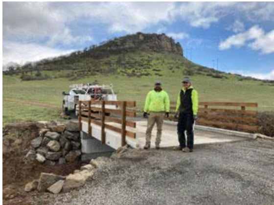
Left: An irrigation ditch bridge at SOLC's Harry and Marilyn Fisher Preserve at Pompadour Bluff, whose unstable footings would not support vehicles necessary for recreation, stewardship or fire safety. Right: The replacement pre-cast bridge with 60,000 pound capacity.
