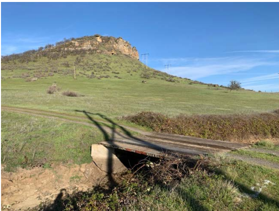
Left: An irrigation ditch bridge at SOLC's Harry and Marilyn Fisher Preserve at Pompadour Bluff, whose unstable footings would not support vehicles necessary for recreation, stewardship or fire safety. Right: The replacement pre-cast bridge with 60,000 pound capacity.
