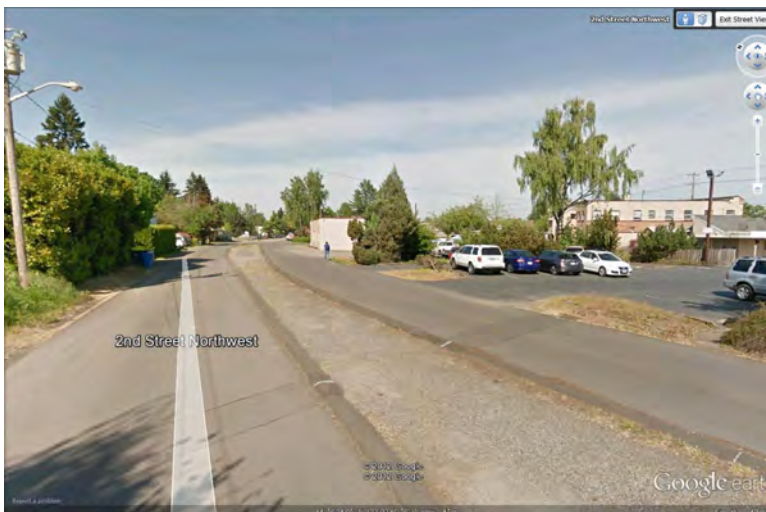
Figure 5: Second Street looking northeast toward downtown
