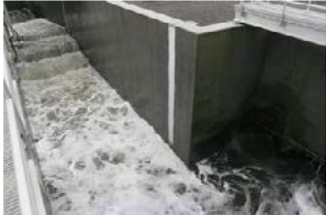
Treated water flows through the outfall into the Willamette River at Willow Lake Water Pollution Control Facility. (KOBBI R. BLAIR | Statesman Journal)
