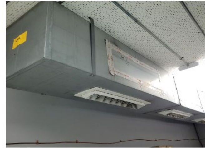
Server room has ad hoc duct work moving air around the room to keep space cool, but with this comes the added need for dust mitigation and dehumidifiers.
