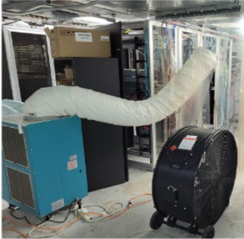
ITC South, current server room, being cooled by added fans and dehumidifiers
