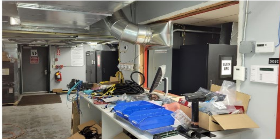
Server room has ad hoc duct work moving air around the room to keep space cool, but with this comes the added need for dust mitigation and dehumidifiers.
