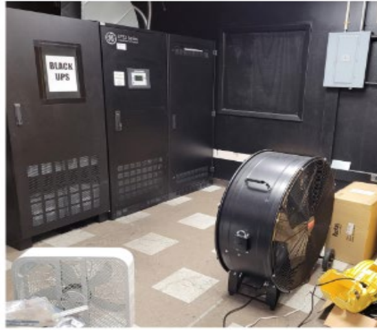
ITC South, current server room, being cooled by added fans and dehumidifiers
