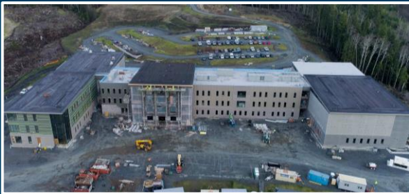
Seaside High School Construction Seaside, OR
