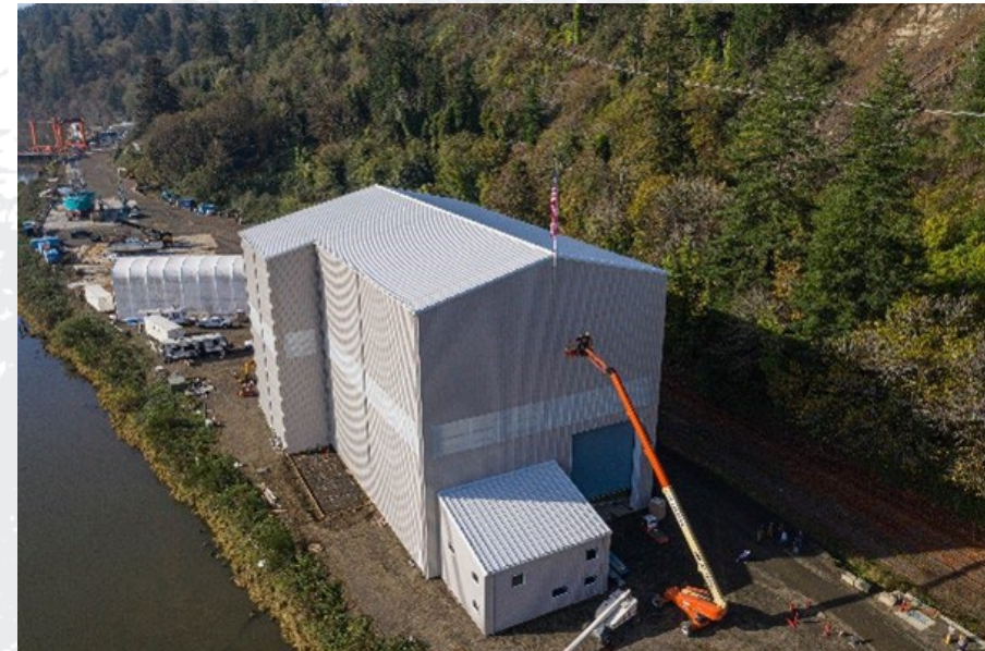
Port of Toledo Redesigned Maritime Maintenance Facility
