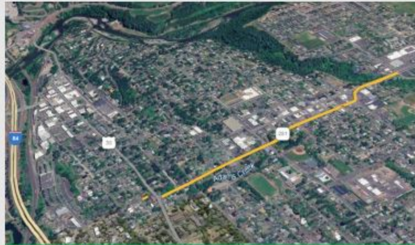
OR 281, Hood River – $30.6 million From 13 th & Cascade avenues to Pacific & 12 th avenues.
