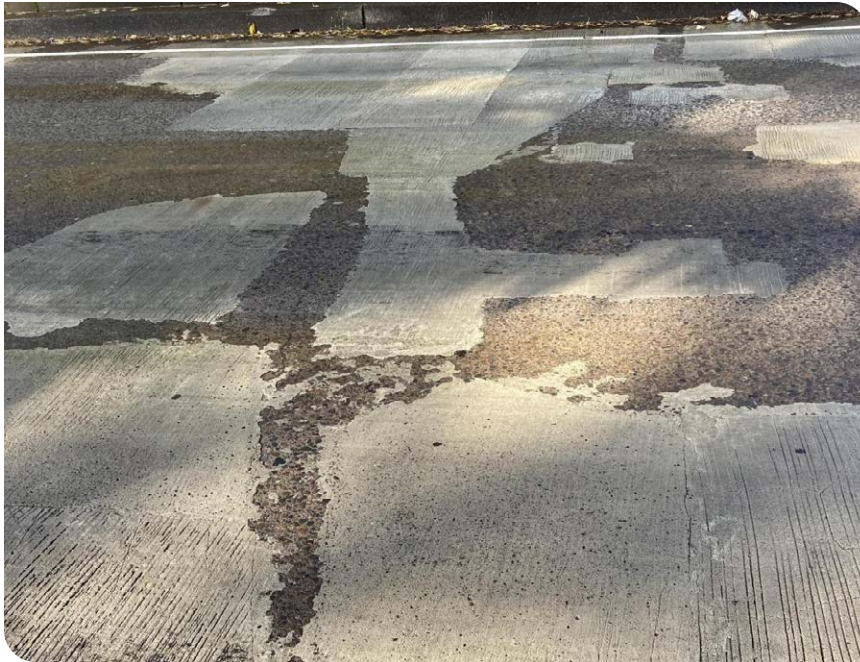
Oregon 18, South Yamhill River Bridge.
