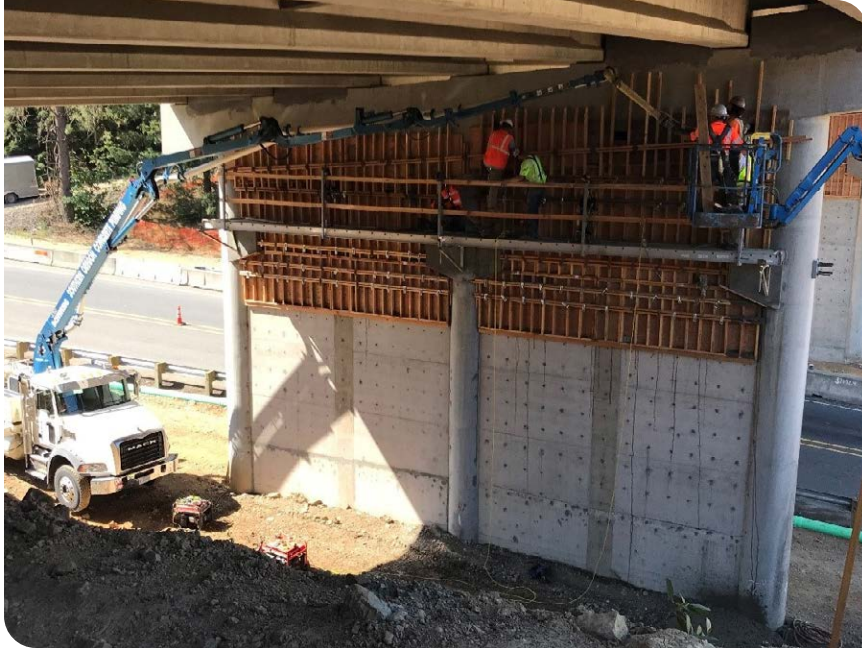
Bridge support strengthening on Southern Oregon Seismic Bridge Retrofit Project.
