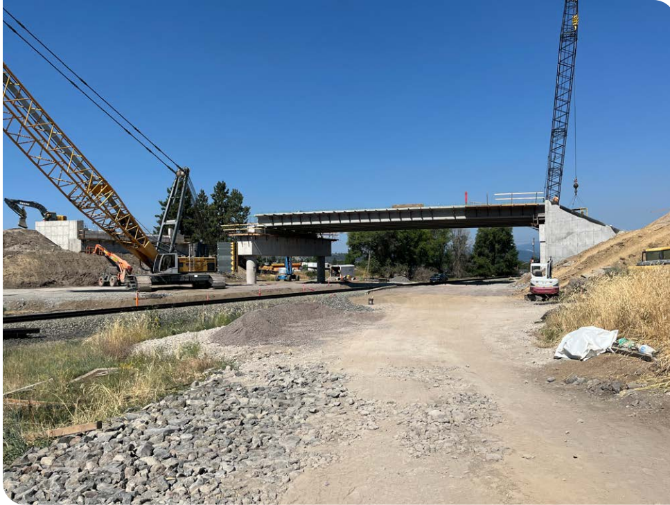
Pelican City Bridge— Placing precast concrete girders.
