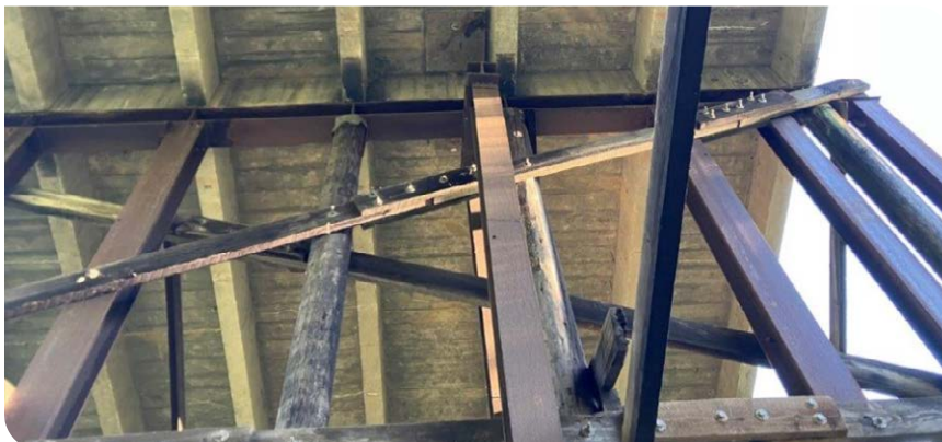
Hess Creek Bridge, Newberg, Oregon.
