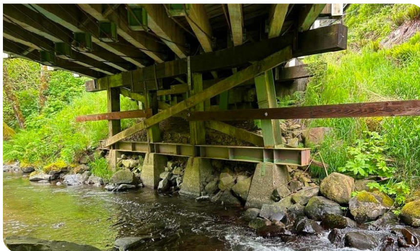
Bear Creek Bridge, Oregon 130.
