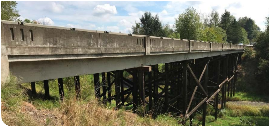
Hess Creek Bridge, Newberg, Oregon.
