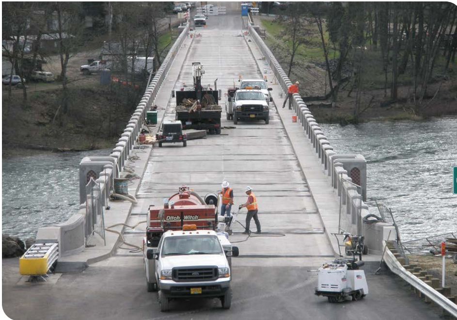
Winchester Bridge over the North Umpqua River (Roseburg, OR) – Bridge Rail and Widening work (2008).
