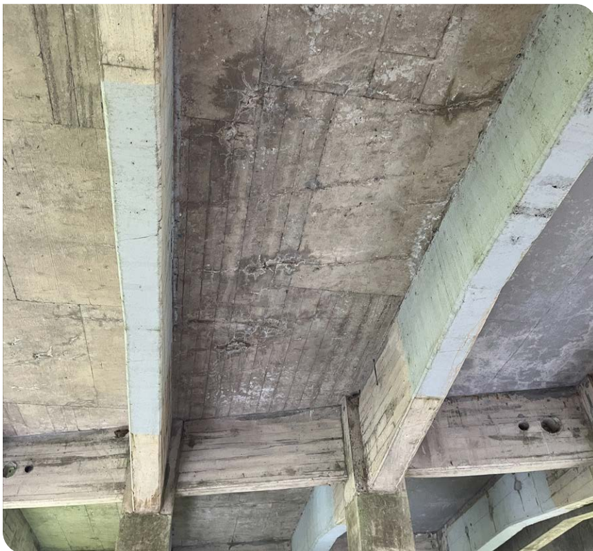
Elk Creek Bridge, northbound I-5.
