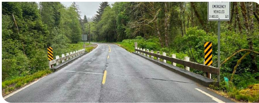
Bear Creek Bridge, Oregon 130.
