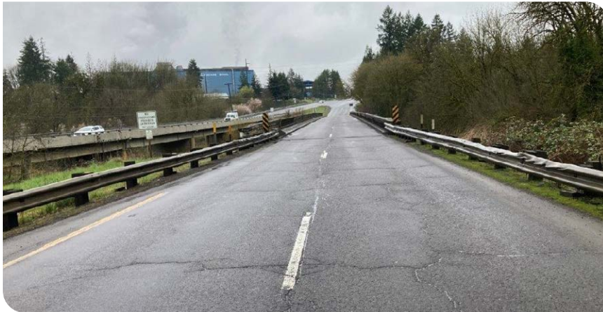
Oregon 99W southbound Yamhill River Bridge.
