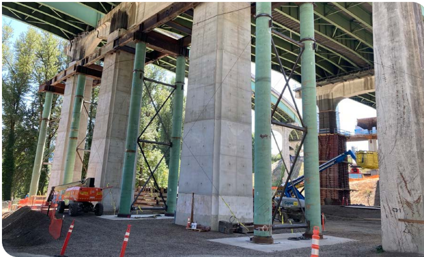
Abernethy Bridge: Enlarging existing bridge columns.
