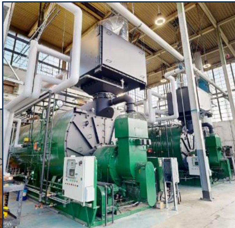
OSP Boiler Replacement Project
