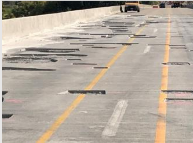
I-84: Snake River Bridge Deck Repairs
