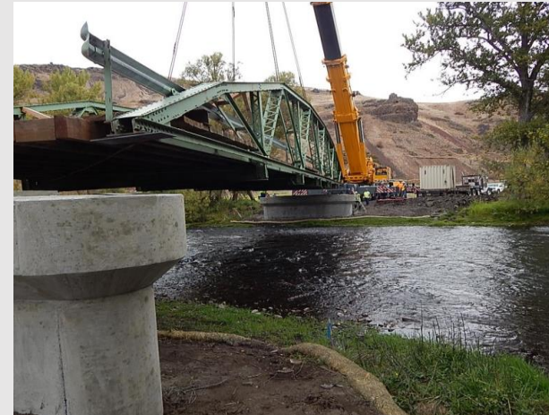
Deer Creek Rd: Wallowa River Bridge
