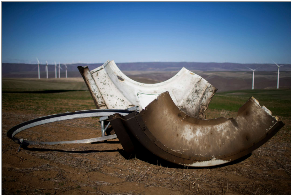
Pieces from a damaged Vestas V82 wind turbine at Biglow Canyon. PGE told regulators a metal frame and pieces of fiberglass fell off the turbine in April 2021. Wind technicians later lowered the turbine’s nose cone and spinner frame to the ground, where they were left for a year.
