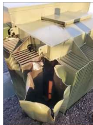
PGE has experienced 10 transformer failures at Biglow Canyon that have collectively leaked 3,000 gallons of mineral oil to the ground surrounding turbines and caused two fires. Pictured above, pad-mount transformers sit in cabinets below each turbine at Biglow Canyon.
