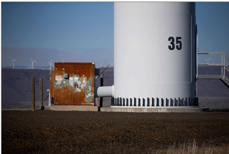
PGE has experienced 10 transformer failures at Biglow Canyon that have collectively leaked 3,000 gallons of mineral oil to the ground surrounding turbines and caused two fires. Pictured above, pad-mount transformers sit in cabinets below each turbine at Biglow Canyon.
