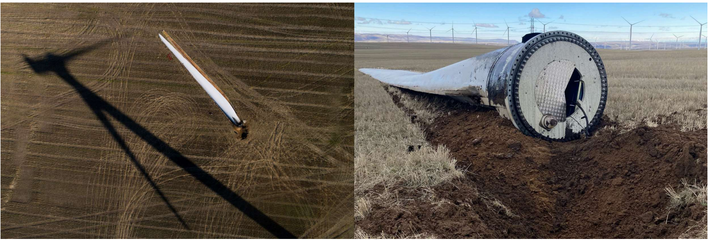
On Feb 1, turbine 71 at Portland General Electric's Biglow Canyon wind farm threw an eight-ton blade 100 yards into a nearby field, plowing a deep furrow in the ground where it landed. (Left, Dave Killen, right courtesy Kathryn McCullough)
