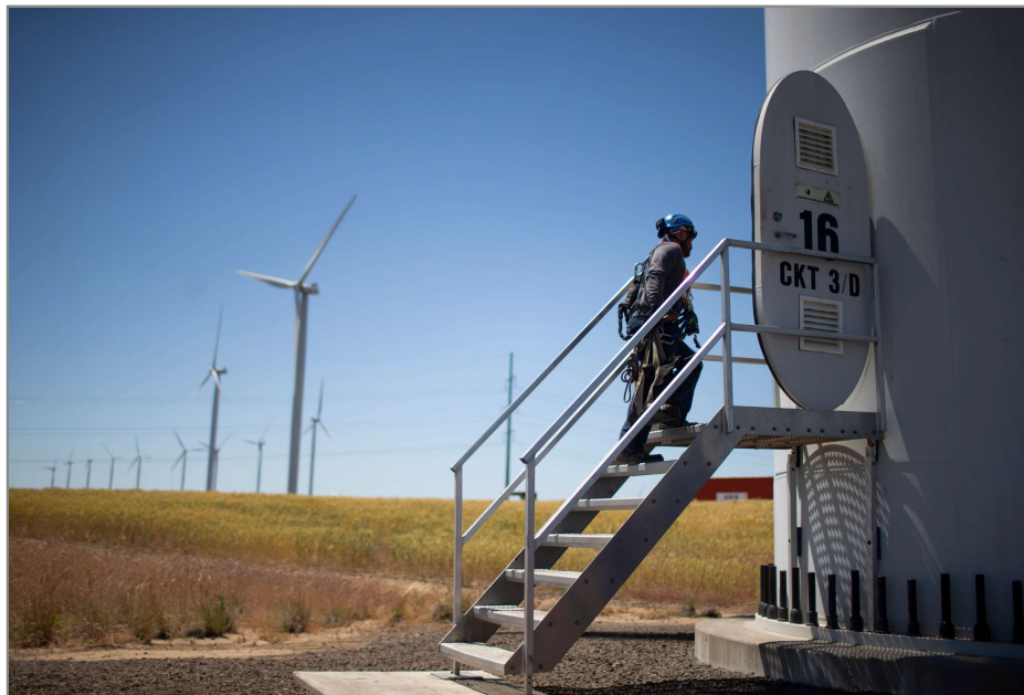
A wind technician enters a Vestas turbine at PGE's Biglow Canyon wind farm. The project's 76 Vestas turbines are now 15 years old, about halfway through their depreciable life. PGE is already considering replacing them.
