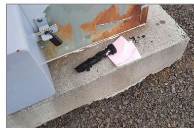
A broken blade bolt found under a wind turbine at Biglow Canyon wind farm by a worker delivering fertilizer in late January. A day or two later, the turbine threw an eight-ton blade into a nearby field. (Courtesy Kevin Massie)
