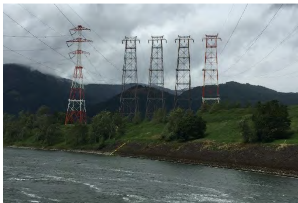
Transmission towers at the Bonneville Dam.
