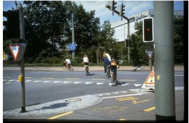
Figure 14. Left-turn from a cycle track on the right via bicycle-signal phase in Winterthur, Switzerland
