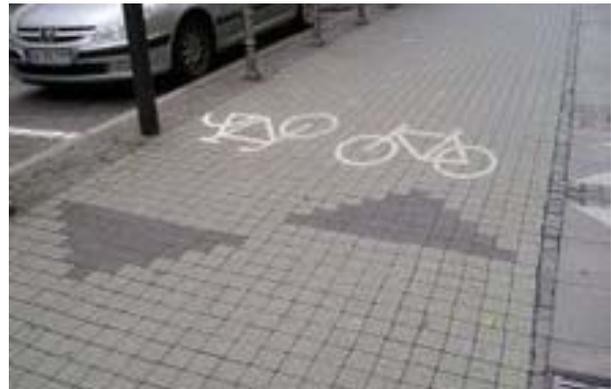
Figure 19. Directional markings on cycle track
