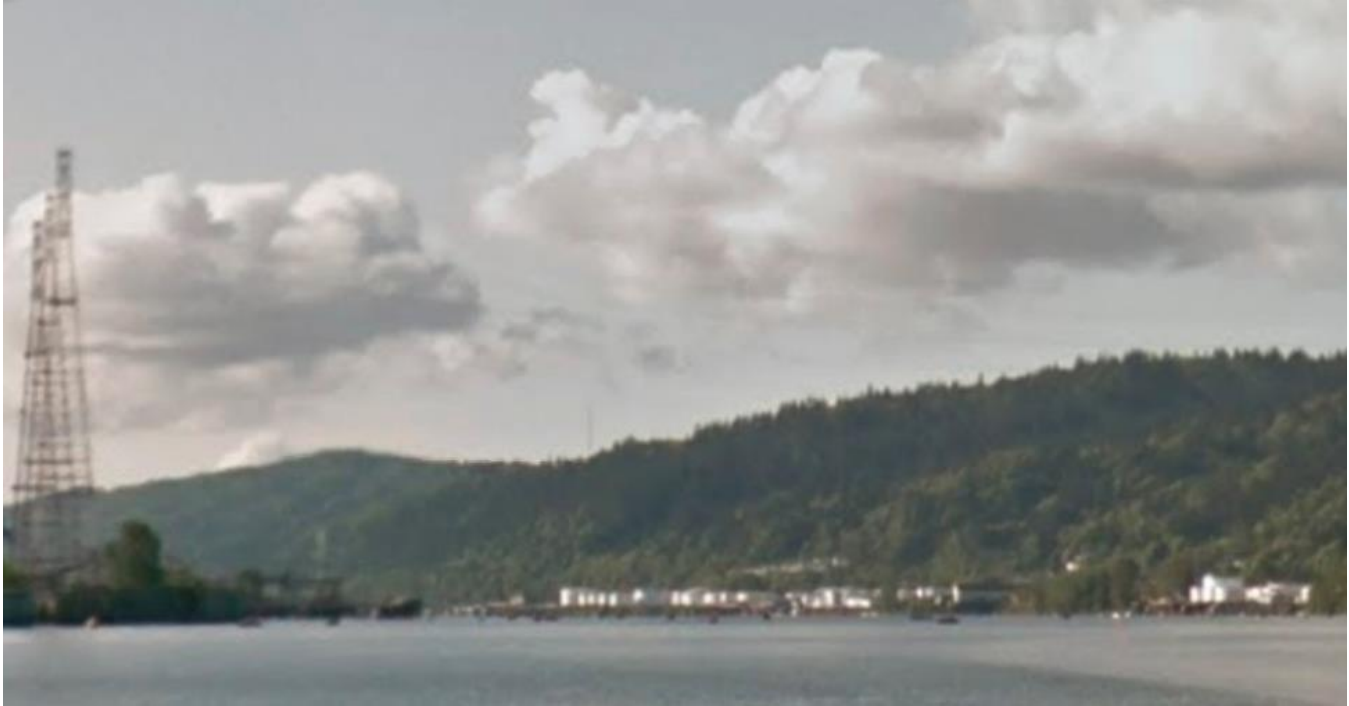
Portland's precarious Linnton fuel storage tanks located upriver 2 mi from Sauvie Island
