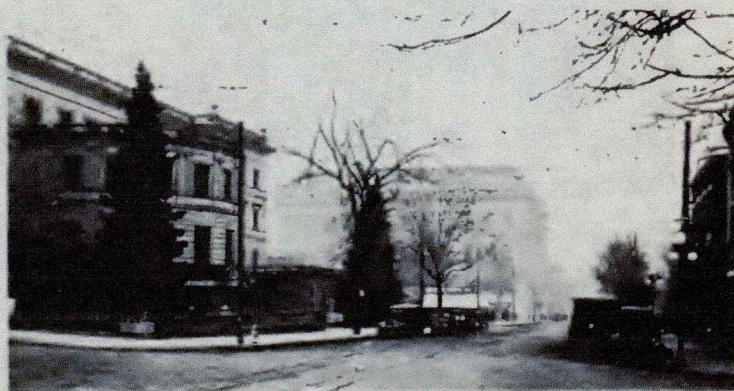
INTERURBAN CENTERS AND CARS. Junction at Fourth and Jefferson Streets, Portland. Southern Pacific line
