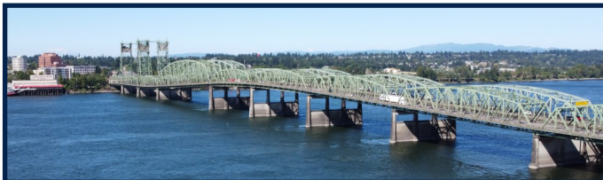
105-year old I-5 Bridge
