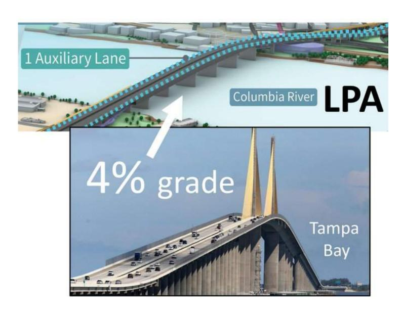
Tampa Bay Bridge is the country's steepest Interstate bridge with no curves on its -4% grade. It has little truck traffic.
