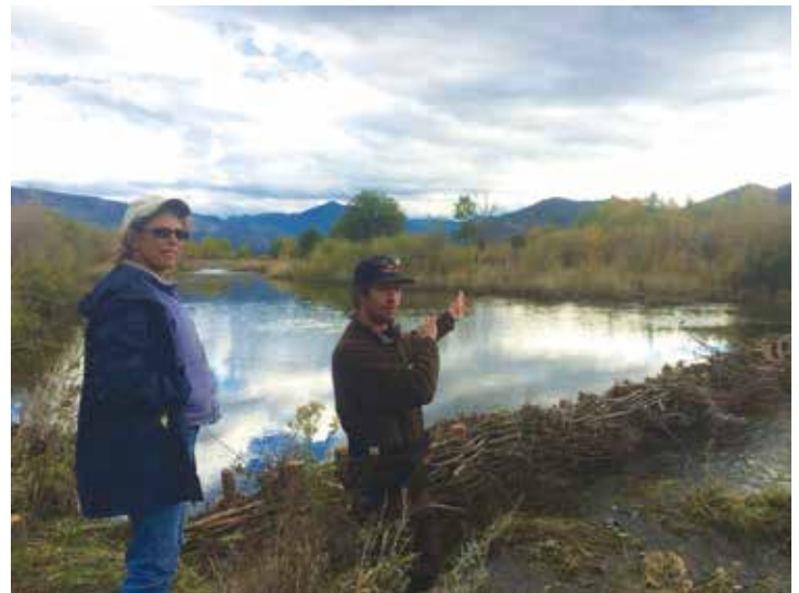
Betsy Stapleton and Peter Thamer standing near a newly installed beaver dam analogue on the Scott River. (Photo: Scott River Watershed Council)
