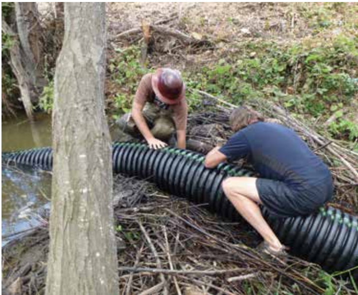
Kevin Swift (on right) of Swift Water Design installs flow control device for Caltrans in Monterey County. (Photo: Kate Lundquist/OAEC)
