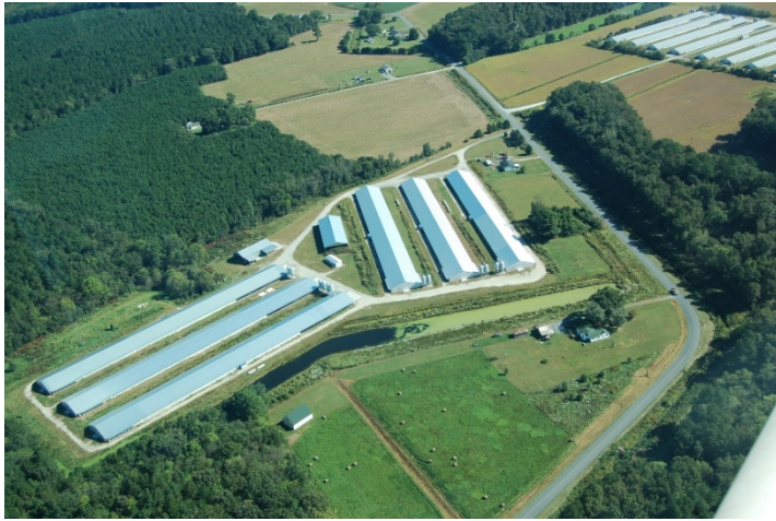
This aerial photo shows Sam Berley's home at bottom right and the six new poultry houses built in 2015 by an adjacent property owner.
