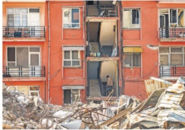
A man walks up the staircase of a damaged apartment complex next to a destroyed building after an earthquake in Samandag, southern Turkey. The author writes that modern building techniques can mitigate the number of deaths.
