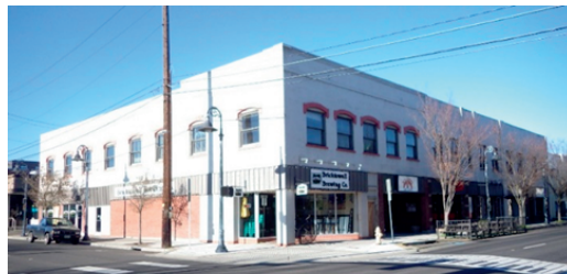
Front elevation, prior to rehabilitation
