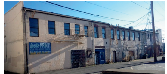
Back elevation, prior to rehabilitation
