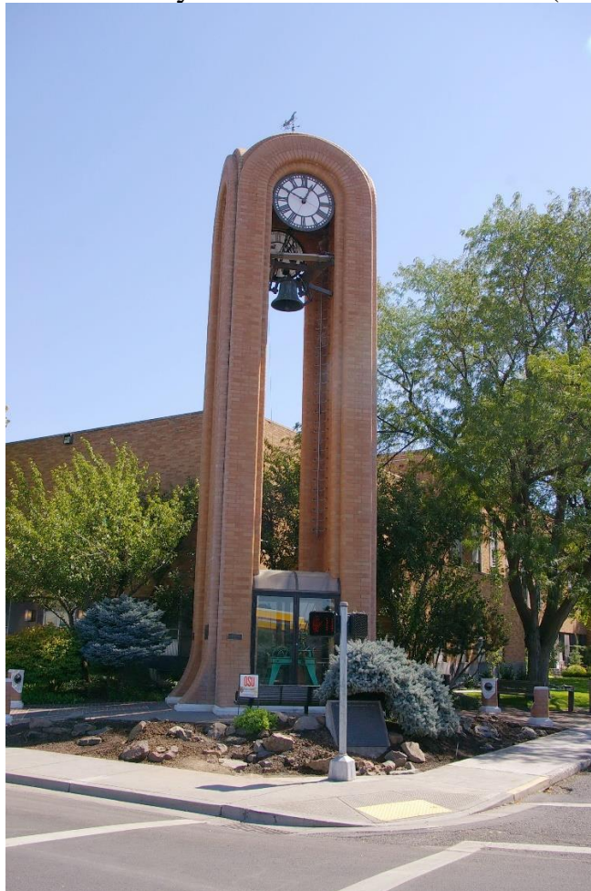
Umatilla County Court House Clock Tower - Pendleton (2012)
