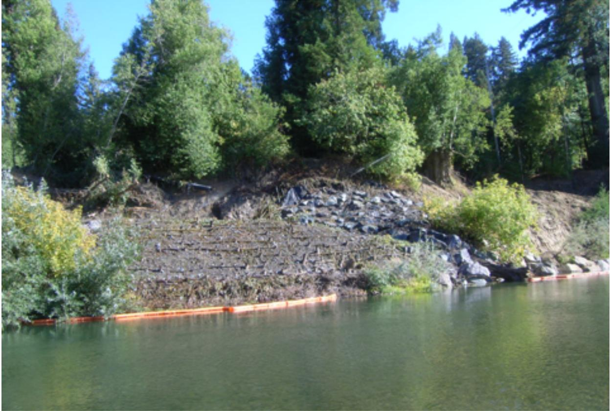
The reshaped section was stabilized with a Live Willow Brush Mattress, pinned down at the toe by a Woven Willow Wall. On the right, another Boulder Wing Deflector.
