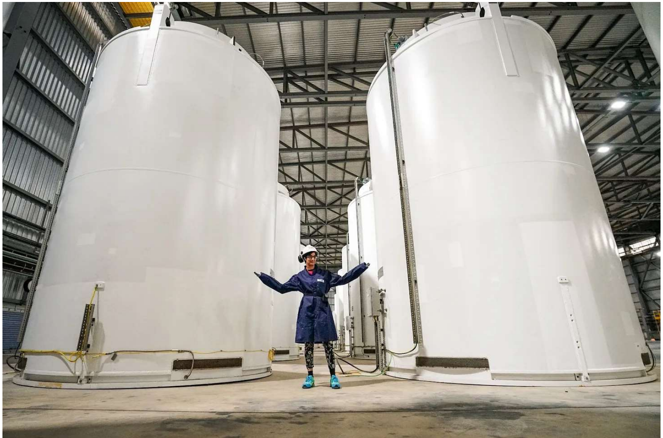
Visiting dry storage casks at Sizewell B in Suffolk, UK
