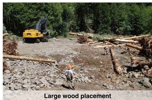
Large wood placement
