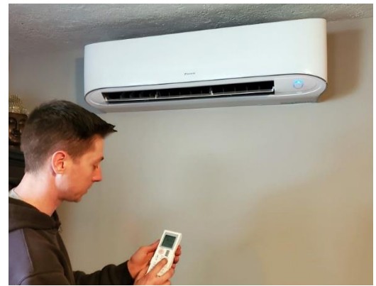
Technologies like ductless heat pumps can support the efficient electrification of buildings.
