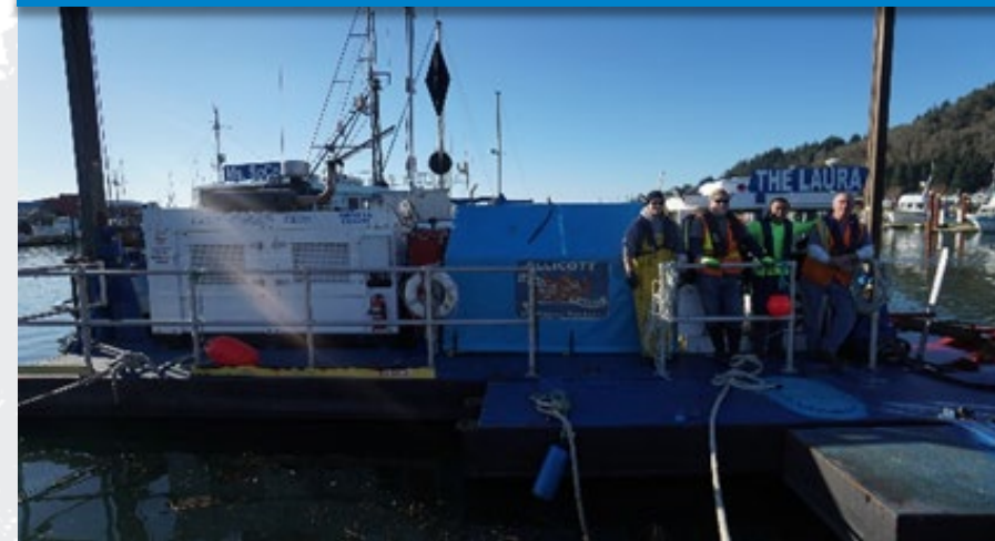
Dredging Project in Coos Bay
