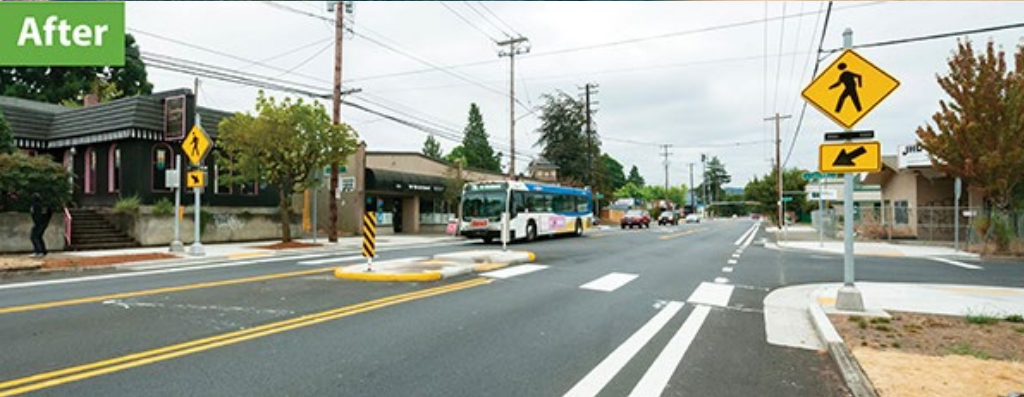
Above: North Lombard Street shown before safety improvements and after, with an RRFB and median refuge island for safer and more visible pedestrian crossings.
