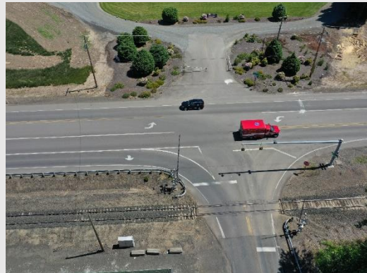
U.S. 20: Safety Upgrades, Albany to Corvallis
