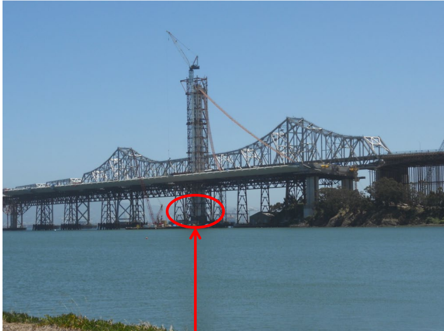
525ft tall tower for the Oakland Bay bridge
