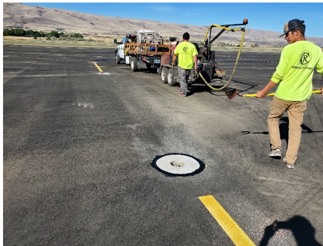
2019 – North Apron Reconstruction Total Project Cost: $1,939,144 ODA COAR Grant: $150,000
