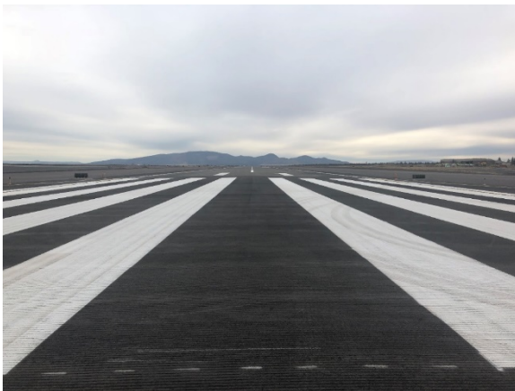
2018 – Runway Rehabilitation project Total Project Cost: $9,826,455 ODA COAR Grant: $145,431
