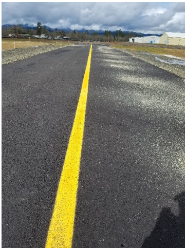
2017 – West Side Taxiway Project Total Project Cost: $75,000 ODA COAR Grant: $67,245
