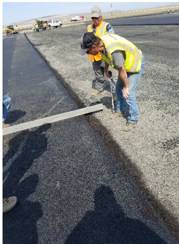
2017 – Apron Construction Total Project Cost: $573,528 ODA COAR Grant: $51,617
