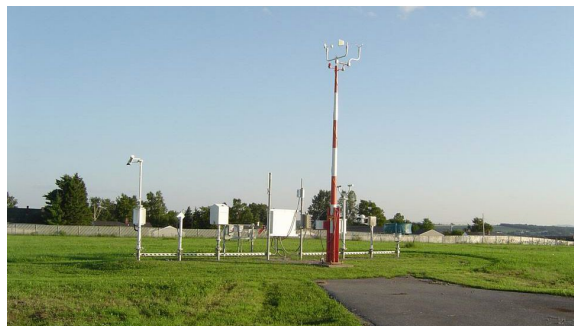
2020 – AWOS Replacement Total Project Cost: $350,000 ODA COAR Grant: $150,000
