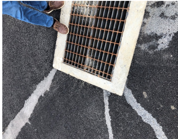
2019 – Ramp Rehabilitation Project Total Project Cost: $1,000,000 ODA COAR Grant: $75,000
