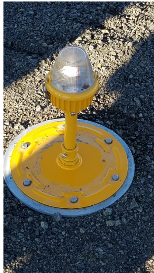
2017 – Runway Lighting Total Project Cost: $140,000 ODA COAR Grant: $133,333
