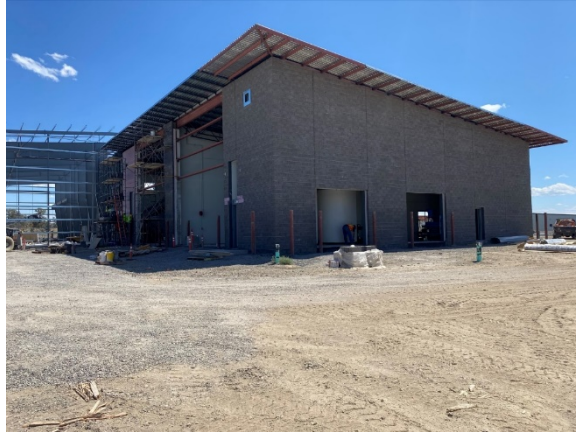
2019-Snow Removal Equipment Building Total Project Cost: $2,684,385 ODA COAR Grant: $102,901
