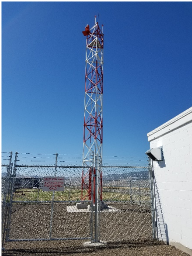
2017 – Airport Beacon and Beacon Tower Improvements
