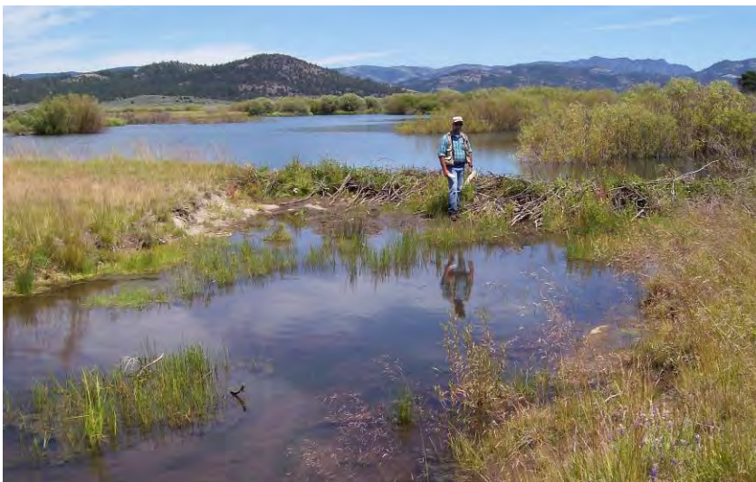
Figure 13: At the Red Clover - McReynolds Project, flow had cut through a plug shortly after construction due to damming of the designed base flow channel. Beaver subsequently dammed the cut at the plug so that base flow elevation is maintained upstream of the plug. (Photo: Joe Hoffman)
