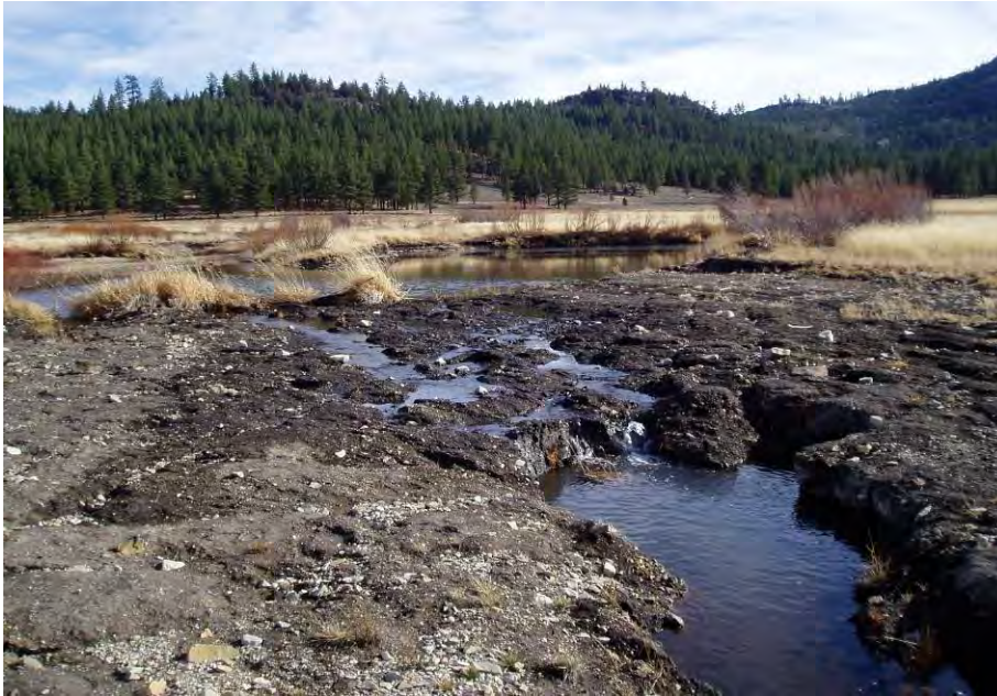
Figure 11: Excessive flow over this plug on Last Chance Creek at Jordan Flat during the 2006 floods caused the base flow to be diverted over the plug. Excessive flow was due to unforeseen dynamics between Last Chance Creek and a tributary stream. A berm was constructed and the problem corrected in 2007. Excessive flow over plugs could headcut through the entire plug, lowering the upstream pond elevation to the elevation of the downstream pond and essentially doubling the head on the next upstream plug. (Photo: Joe Hoffman)
