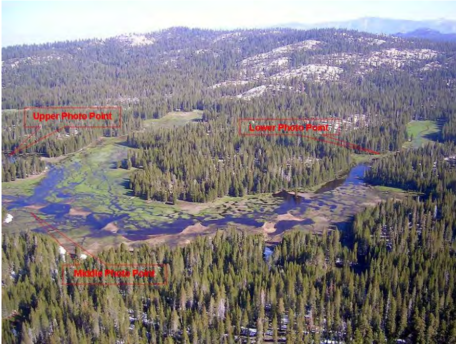
Figure 12: Big Meadows Pond-and-Plug Project, Sequoia NF. Project was constructed in fall 2007. Photo taken in spring, 2008 during the first runoff season. (Photo: Wayne Luallen)
