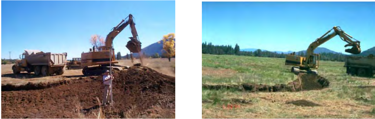
Figure 3 – Sculpting the restored channel in the summer of 1999 (Photos: Rick Poore).
