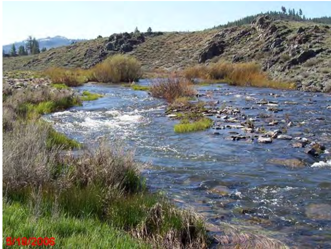
Figure 10: Alkali grade control structure on Last Chance Creek demonstrates the stability of the current design method during a flood in spring 2006. First photo is February 23, 2006, second photo taken on February 28, and third photo in May 2006. Note in the first and third photos that low flows remain in the constructed riffle-pool base flow channel after the flood. (Photos: Jim Wilcox)
