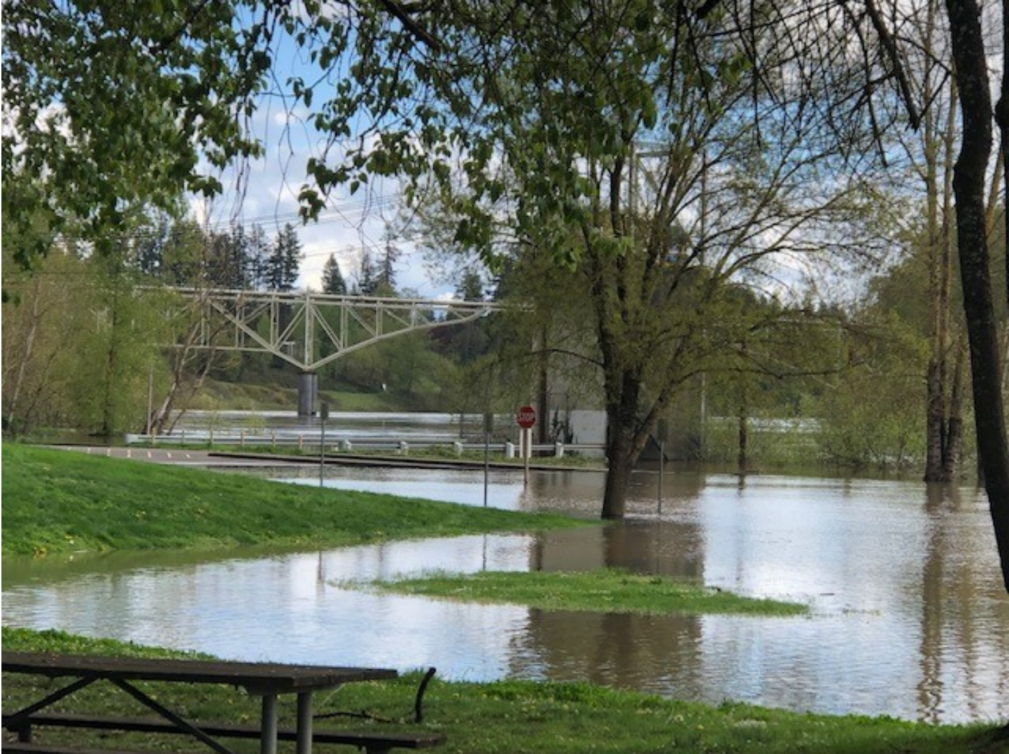
Rogers Landing parking lot and boat ramp – April 12, 2019 (entire parking lot is submerged, with some portions closer to the ramp under 2' of water)
