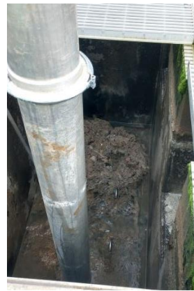
Figure 1- Starting the removal of the material
