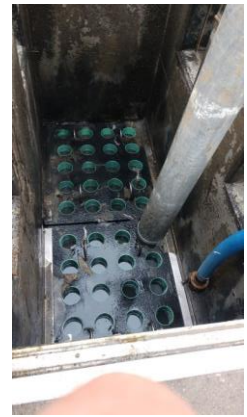
Figure 2- After the removal of the material
