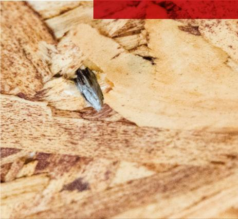
Roofing nails piercing roof decking
