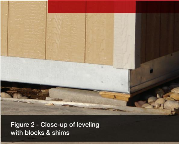
Figure 2 - Close-up of leveling with blocks & shims
