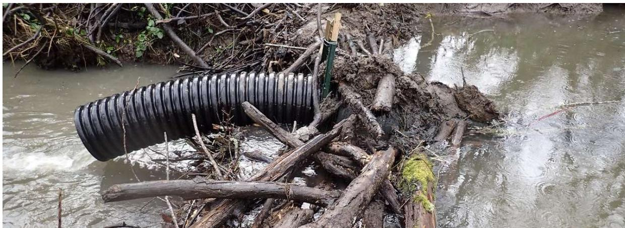
*Outlet pipe of beaver pond leveler installed on Dunawi Creek to help reduce flooding of 53<sup>rd</sup> Street.*
