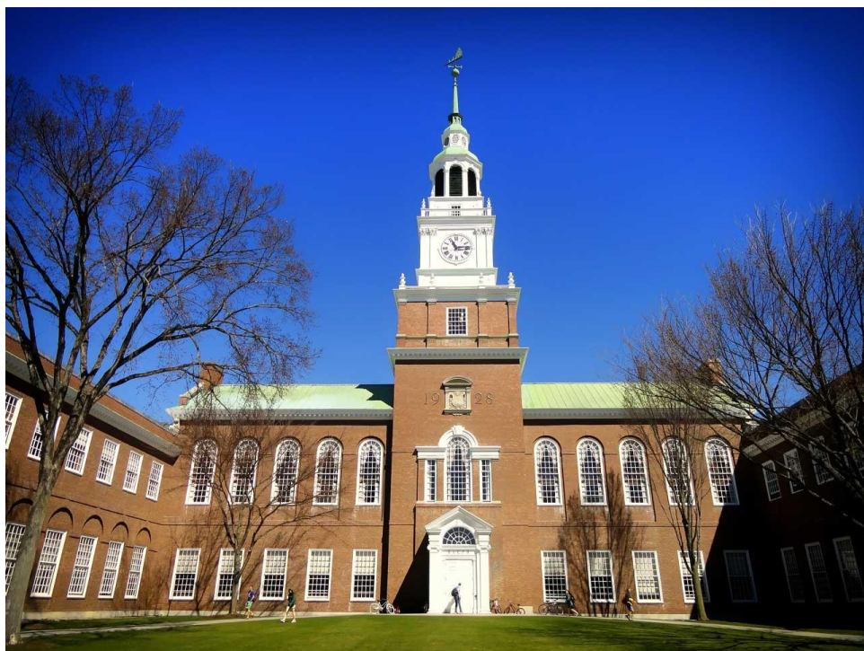
Dartmouth College Campus Library Building (Photo by David Mark , Licensed under Pixabay License )
