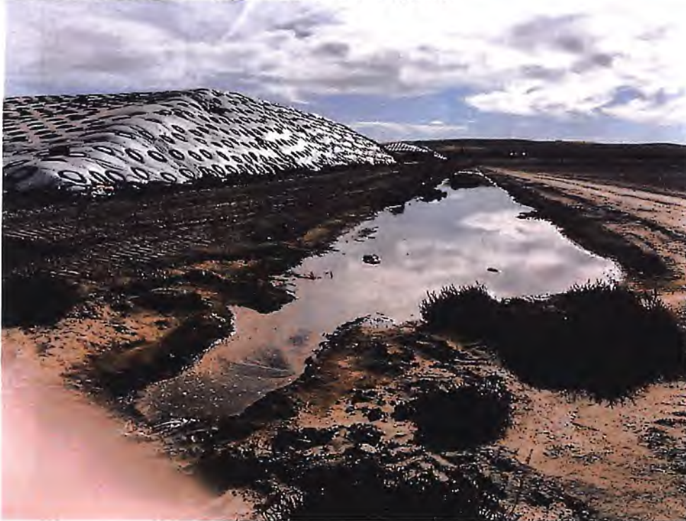
Photo #2: Ponding on swale between silage pad and lagoons.
