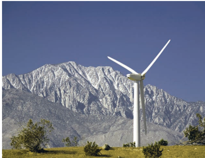
DILLON WIND POWER PROJECT, PHOTO BY IBERDROLA RENEWABLES, INC., NREL 16105
