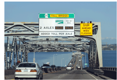
SR 520 Floating Bridge, WA 2
