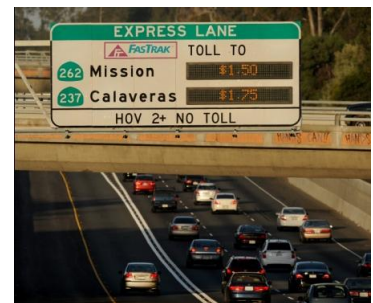
I-680 Express Lanes Alameda County, CA 4
