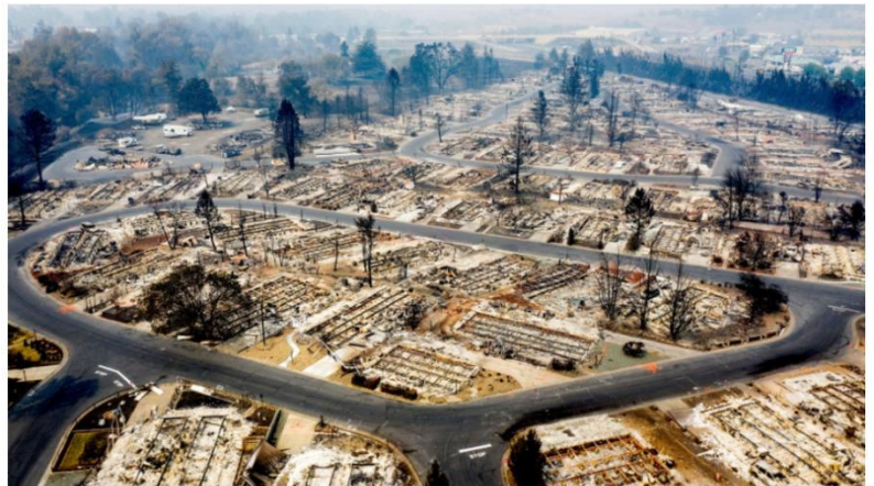
The Bear Lake Estates manufactured home park was among the housing developments destroyed by the Almeda fire. AP Photo/Noah Berger
